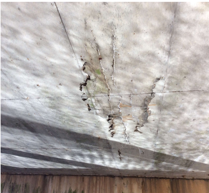
PHOTO 1 Description Typ. Delam & Cracking in Soffit under Long Cracks in Deck.
