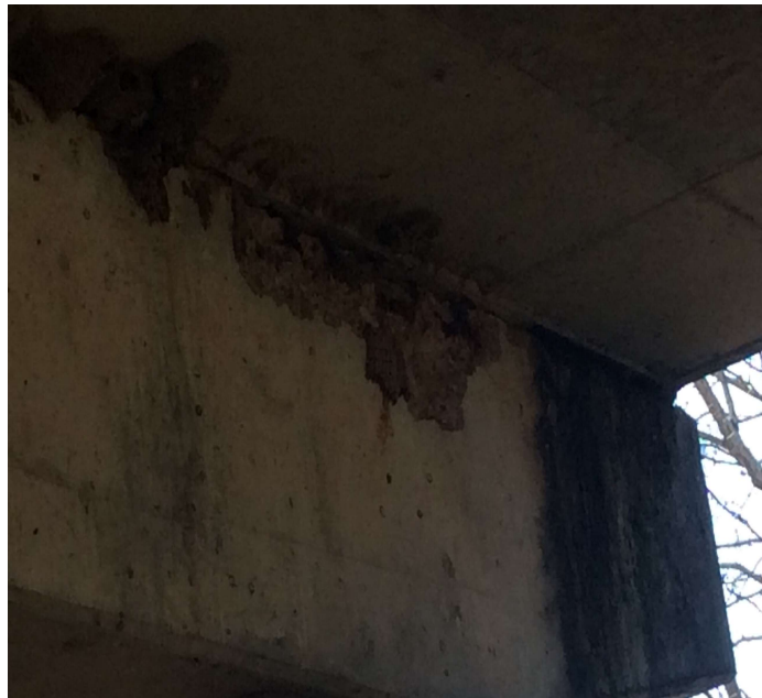
PHOTO 1 Description Minor Delam & Spalling in Bk. Face Cap 4 above Column 3.
