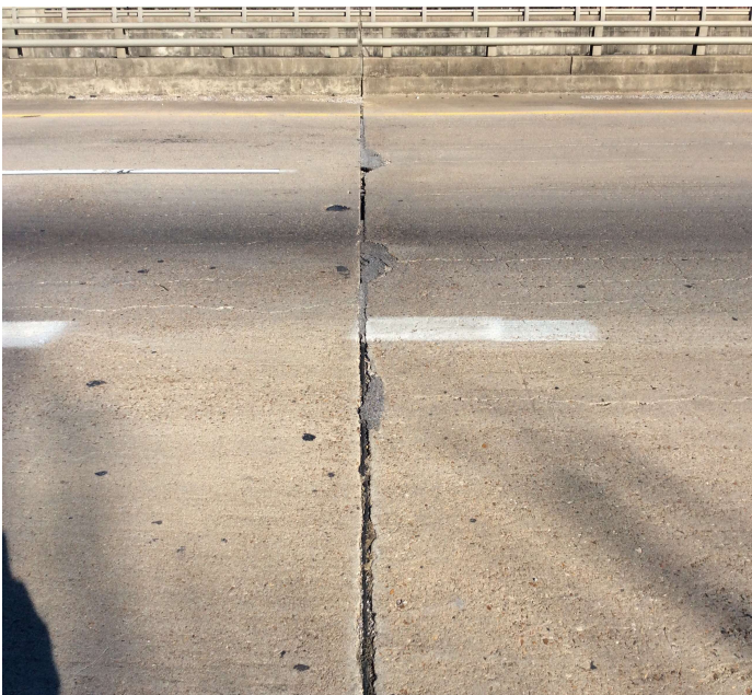
PHOTO 1 Description Typ. Condition of Joints.
