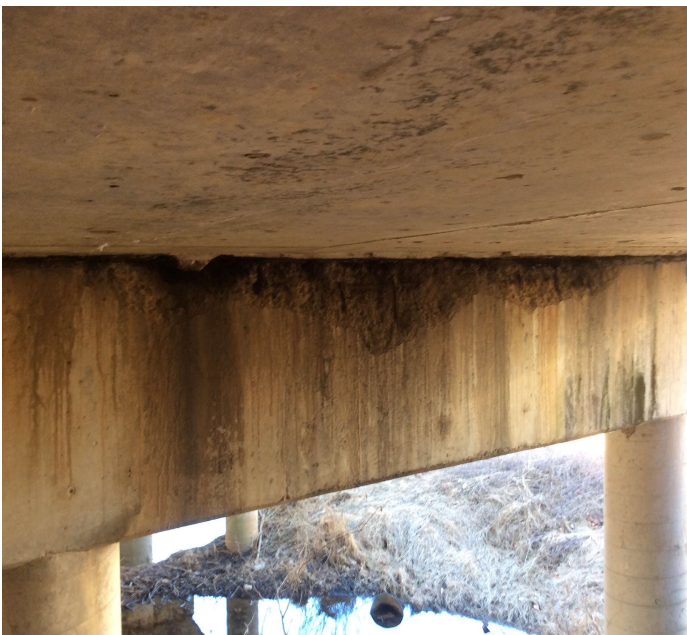
PHOTO 1 Description Delam, Cracking & Spalling W / Rebar Exposed in Ahd. Face of Cap 5.
