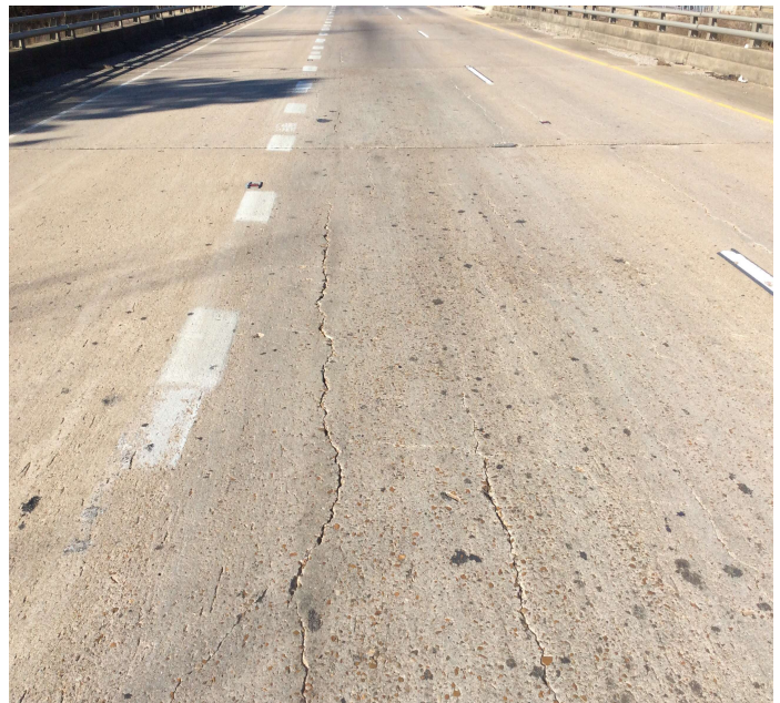
PHOTO 2 Description Typ. Long Cracking in all Spans.
