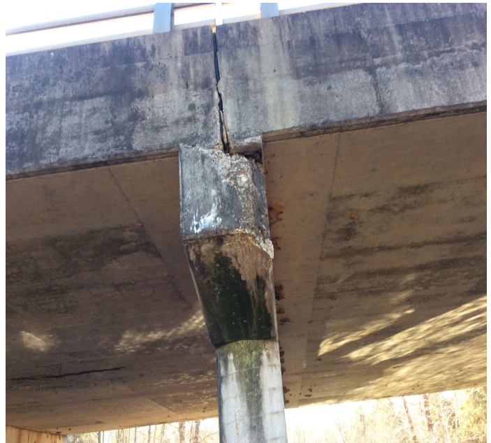
PHOTO 2 Description Delam, Cracking & Spalling in Lt. End of Cap 4 Bk. Side.
